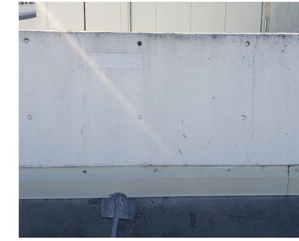
4 TYPICAL PARAPET WALL CRACKS/SPALLS N.T.S.
