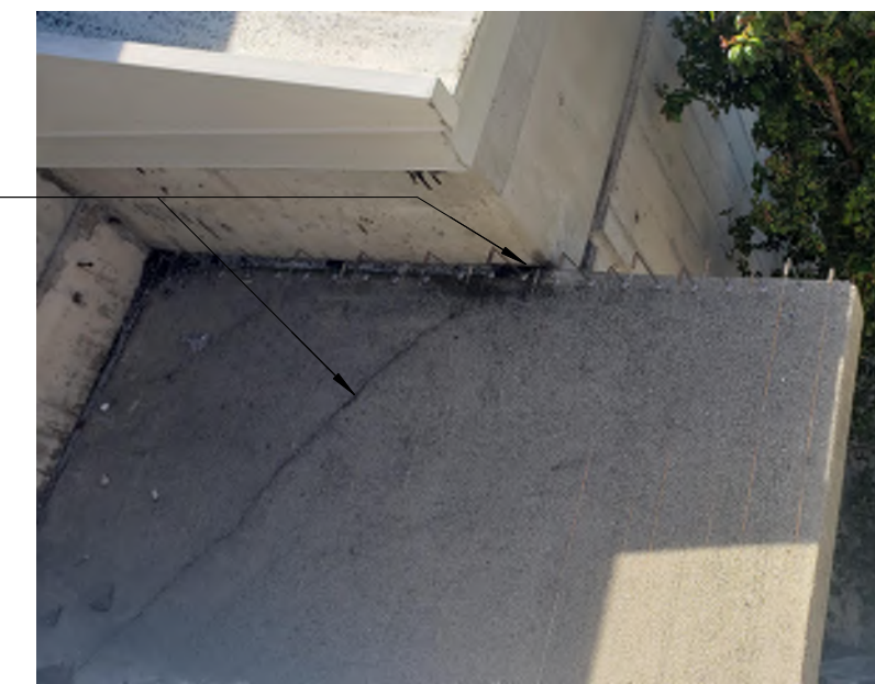
6 TYPICAL EYEBROW CRACKS/SPALLS N.T.S.
