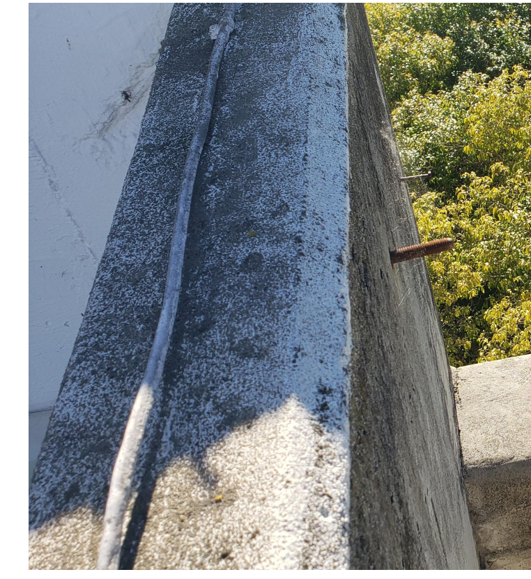
5 TYPICAL PARAPET WALL CRACKS/SPALLS N.T.S.
